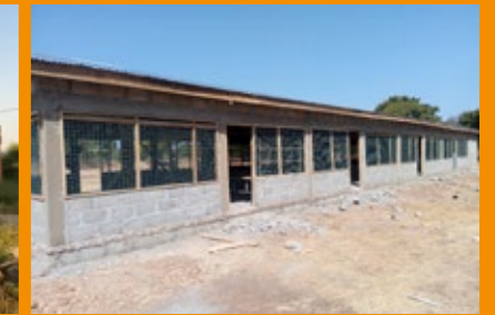
Completed Guinea Fowl farm.
